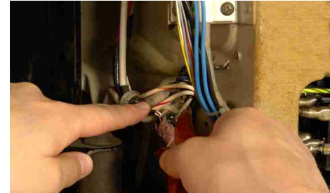
6 Cut connection between thermostat and compressor
