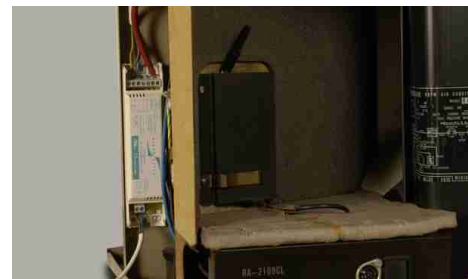
9 Position sensor in supply air stream (example)
