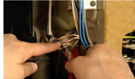
6 Cut connection between thermostat and compressor
