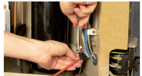
7 Route this switching wire through the AIRCO SAVER (i.e. the AIRCO SAVER is now logically in series with the thermostat). Connect power to the AIRCO SAVER.
