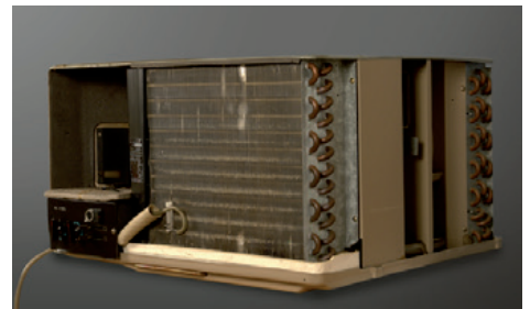
3 Disconnect power & remove covers
