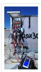
Photo by Joseph A. Garcia / Star staff Testing of an air conditioning unit with the AircoSaver device, which will show its voltage and current, begins. Several air conditioning units were tested before and after they were retrofitted with the AircoSaver device.
